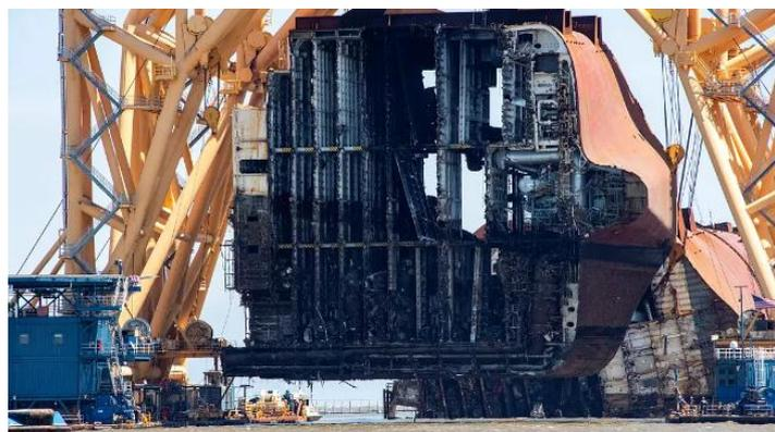
April 28 - On Tuesday, salvors hoisted and removed the engine room section of the grounded ro/ro Golden Ray, loading it onto a deck barge for transport to a recycling facility in Louisiana.
